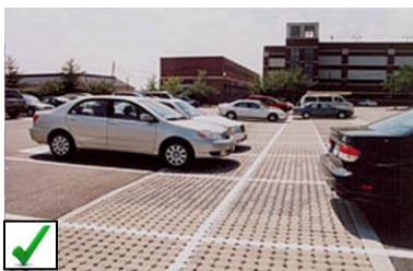
Porous pavers should be utilized in parking areas to help reduce storm water run-off.
