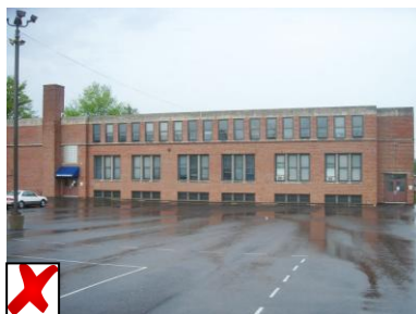
The rear of buildings should be properly landscaped.
