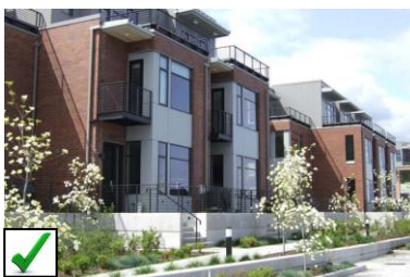
Architectural massing avoids threatening the pedestrian environment by stepping back as height increases.
